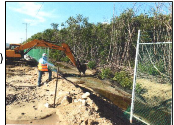
Clearing mangrove channel post Hurricane Bud 2012. (Source: API Manzanillo).
