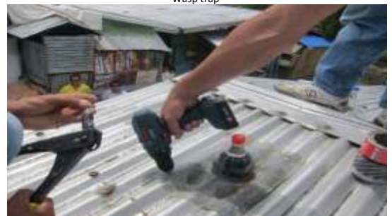
Pop bottles filled with water give light to corrugated steel roof-no electricity
