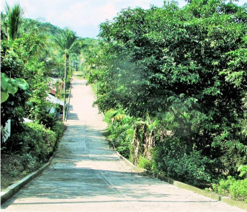
Village street paved
